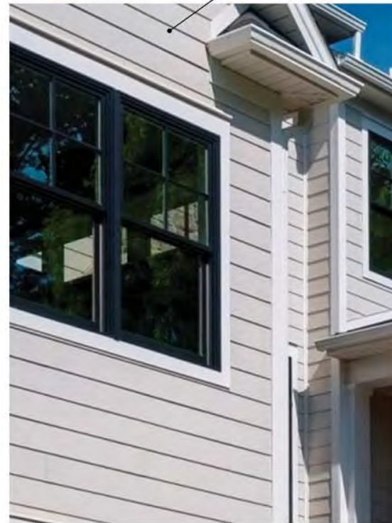
Painted Lap Siding, 4" Exposure
